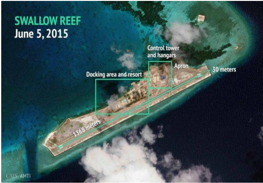
Figure 4: Airstrip on Pulau Layang-Layang (Swallow Reef)
