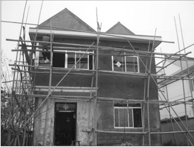
Figure 3 A House in the Building Process (2008)
